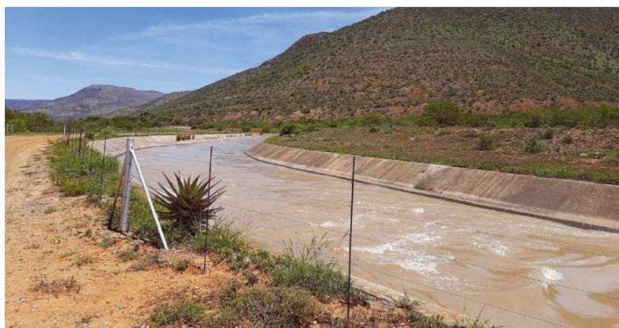
The main canal off the Great Fish River in the Klipfontein area.
