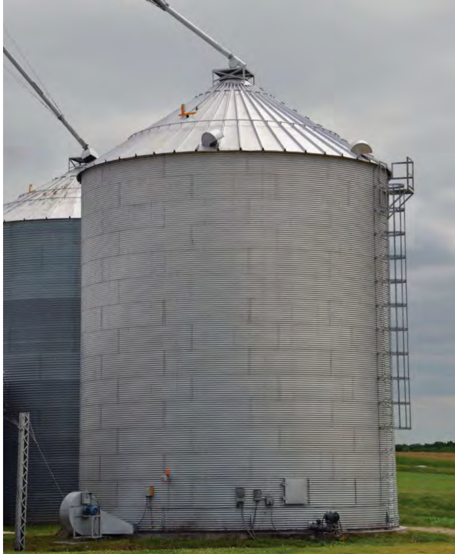
An on-farm grain drying bin can be used for soya beans, but careful consideration must be given to temperature and humidity levels. (Photograph: United Soybean Board)
